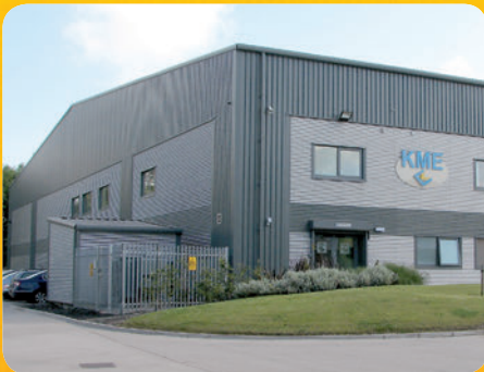
Our new 'state of the art' custom built 42,000sq ft premises.
